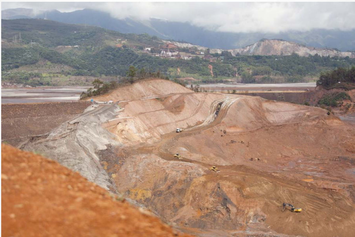
Works on the dam at the Germano Unit
