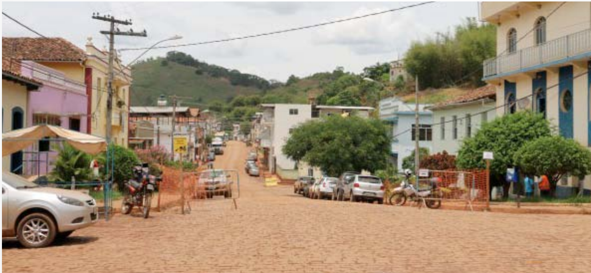
Reclamation work progresses in Barra Longa
