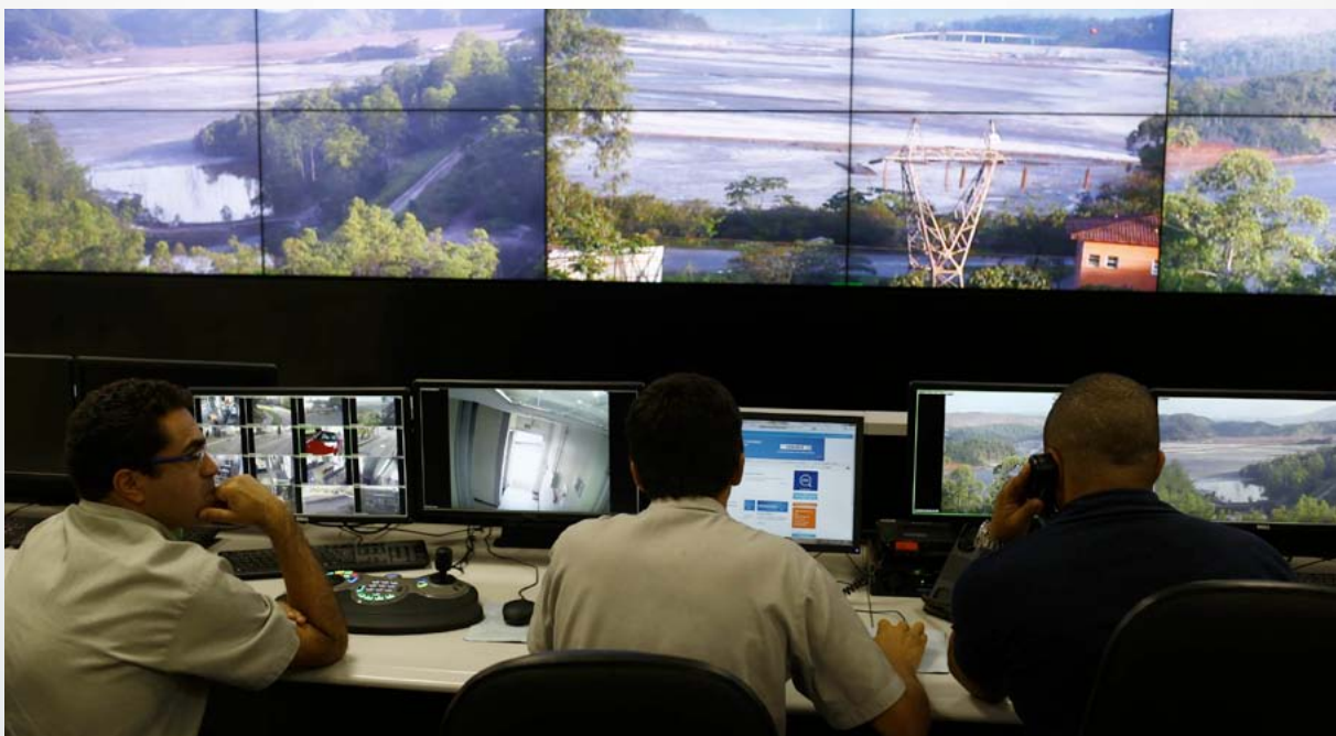
Monitoring room at the Germano Unit
