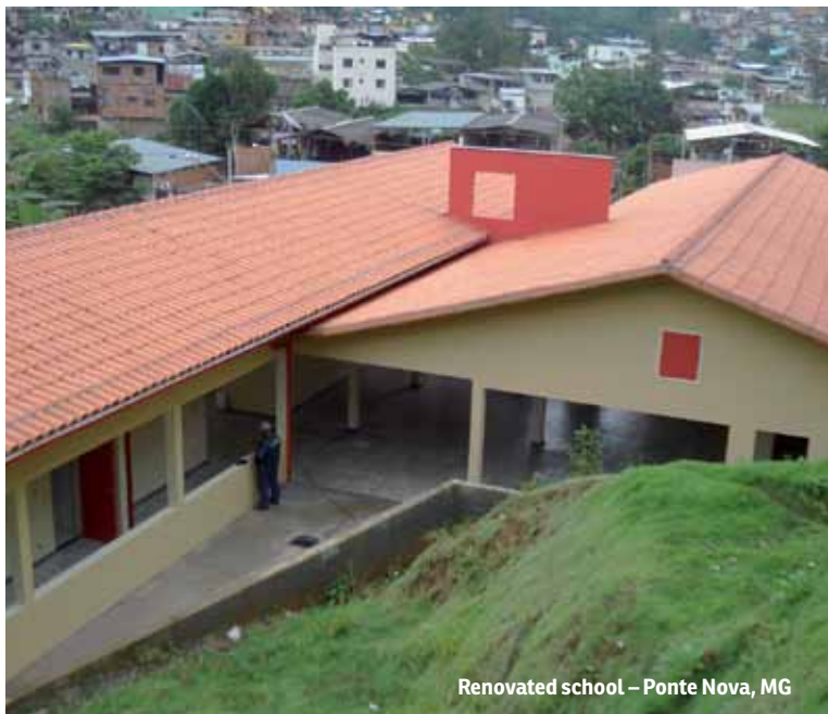
Renovated school – Ponte Nova, MG
