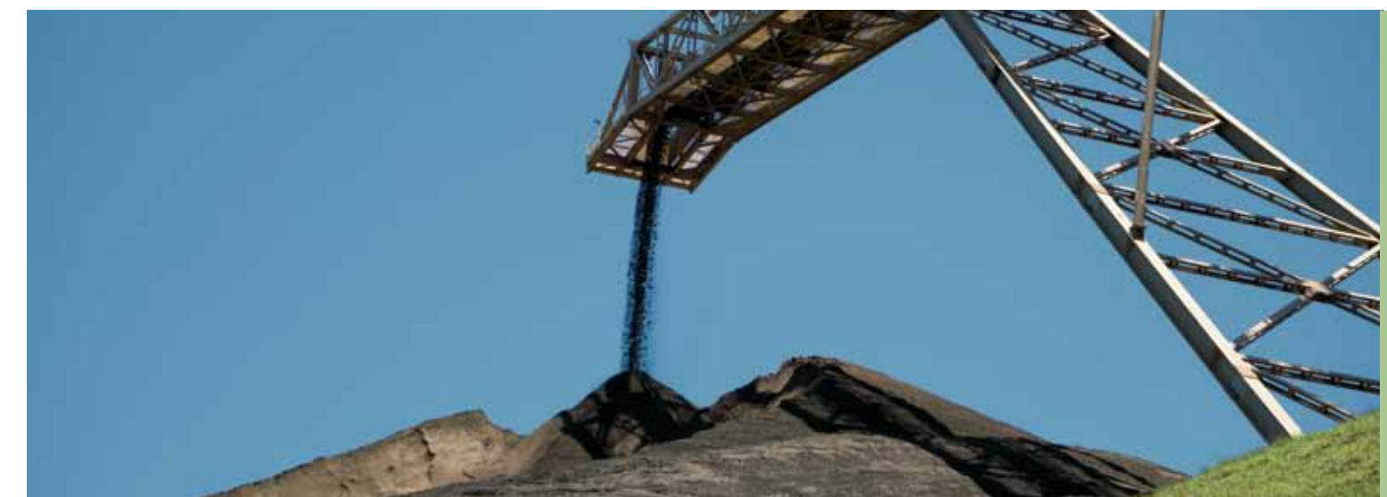
Surge Pile – stacking. Germano-MG
