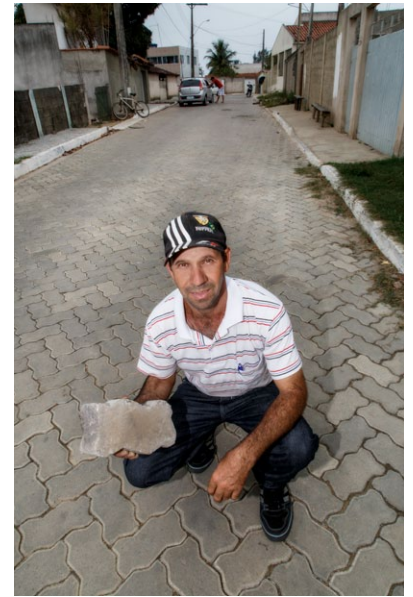
Porto Grande's community received the paving with the interlocking blocks made out of waste.
