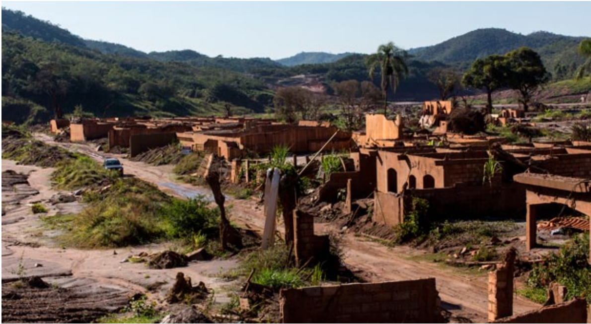
The failure of the dam was an unprecedented environmental tragedy in Brazilian mining
