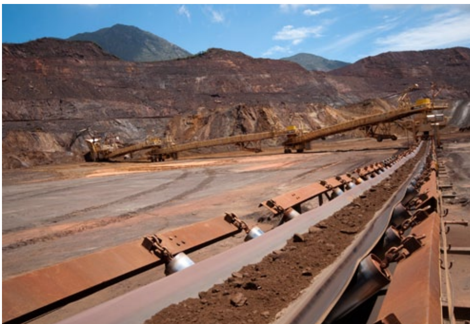
Conveyor belt in the Germano unit
