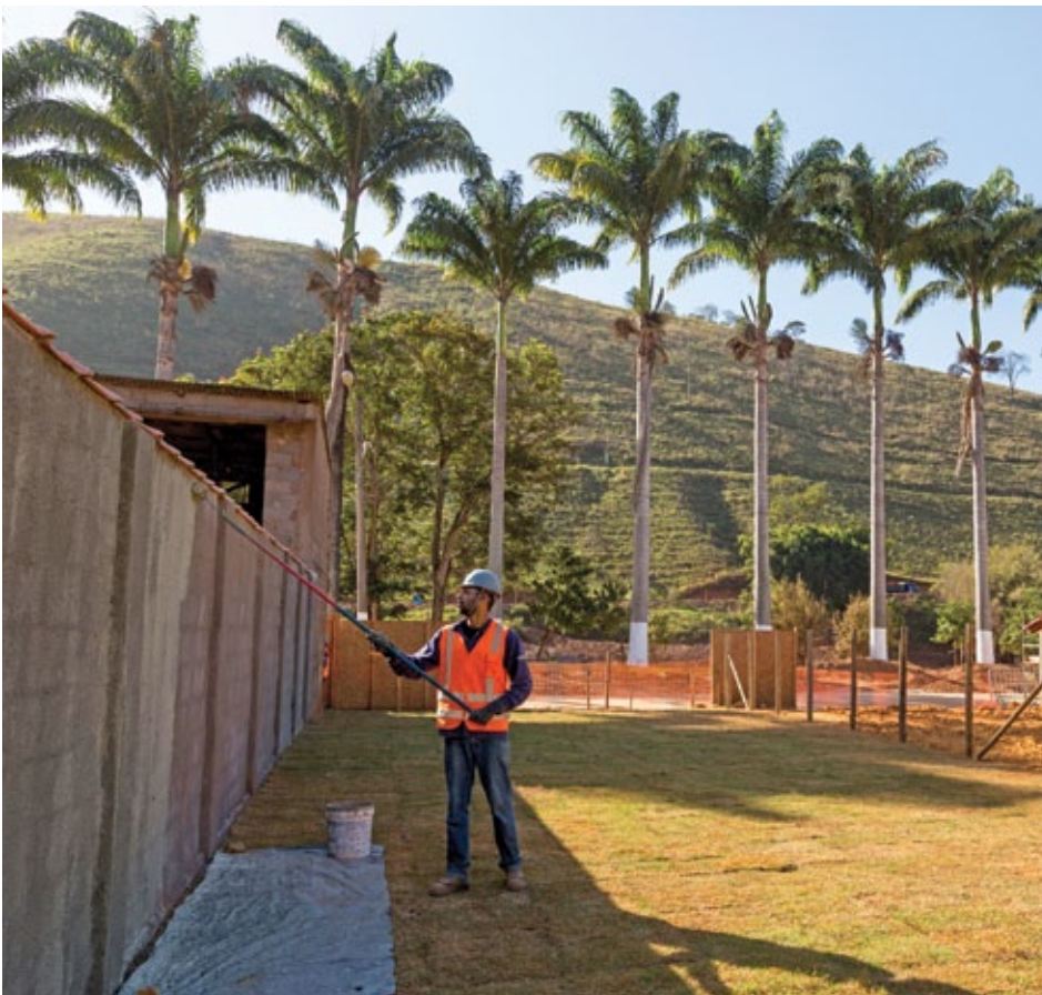
Recovery of backyards in Barra Longa
